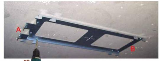
3) Lift the hood to the ceiling bracket. Ensure the holes on top of the motor correspond to the slider fixings on the bracket. Slide in to position
