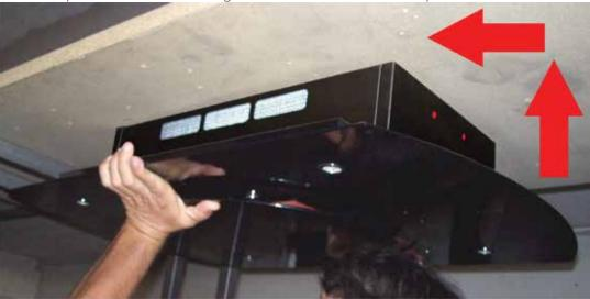
2) Locate the installation holes on top of the motor
