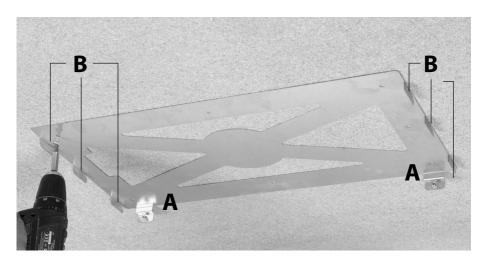
Fix the ceiling bracket to the ceiling in the desired location. We recommends installing the hood with seven wall plugs of minimum Ø10 mm (not included in the kit).
