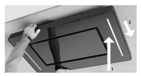
Lift the hood to the ceiling bracket. Ensure the holes on top of the motor correspond to the slider fixings on the bracket. Slide in to position.
